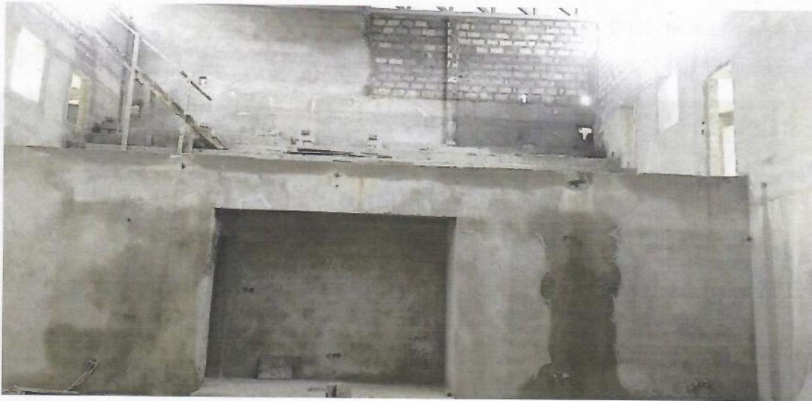
Image 3. Internal view from within the chamber highlighting plastered walls at 65%
