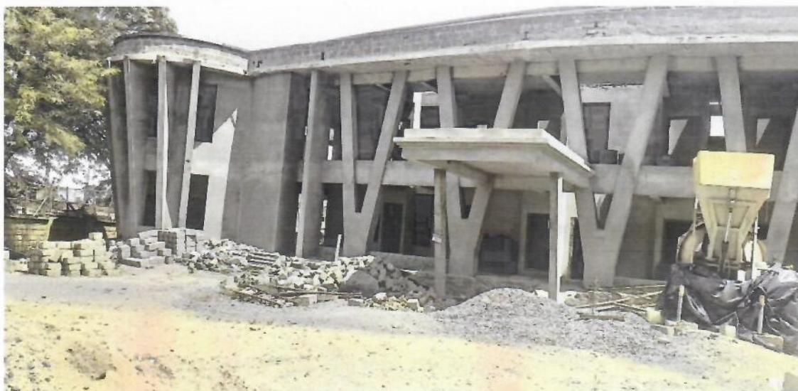
Image 2. View of the project from the site store
